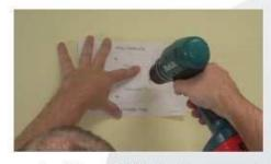
Remove the lid and fit the holder securely to the wall using three screws.
