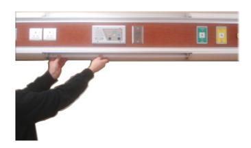
12. Replace lens covers in place using provided screws
